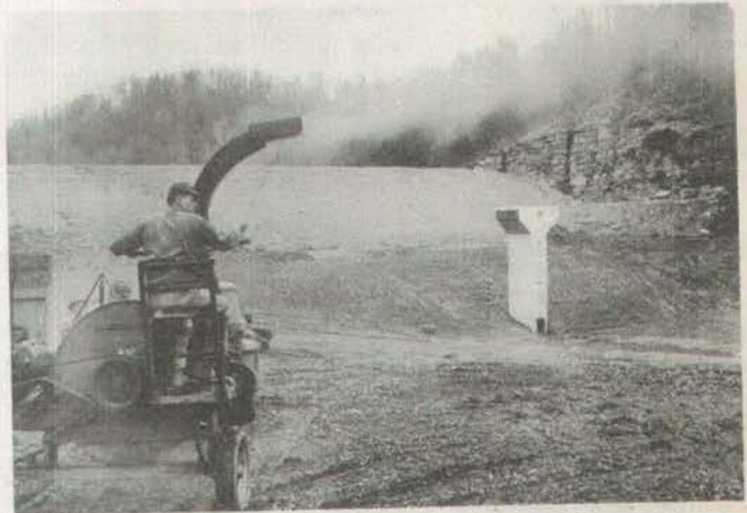
The finishing touch to all watershed dams is a good cover of grass. This machine is blowing mulch on Dam No. 13, Jennings Creek Watershed, Jackson County, Tenn.
