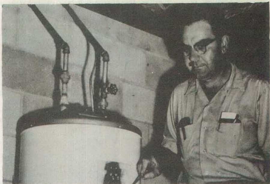
High limit controls are now a requirement in Tennessee on water heaters. This water heater at the home of Larry Benderman, Maury County, is being inspected by Mr. W. L. Butler, Deputy Electrical Inspector.
