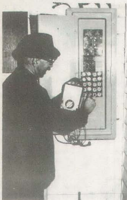
State wiring inspector John S. Fite is shown here inspecting a new 200-amp service entrance installed in an old house.
