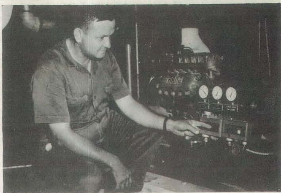
Seen here, inspecting a 30-ton unit of air conditioning at the University of the South Library, Sewanee, is Deputy Electrical Inspector W. B. Lawson. The library has more than 100 tons of cooling capacity for its 116,000 square feet of floor space.
