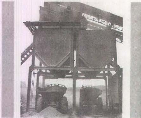
After limestone has been crushed to desired size, it is electrically conveyed to these storage bins, from which huge trucks are loaded for transport of rock to customers.
