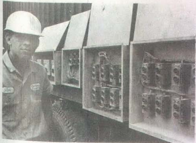
Porter Brown Employee Joe Woodard stands beside the outside pushbutton panels which electrically control all phases of the rock crushing operation. Panel is mounted on 32-foot trailer.
