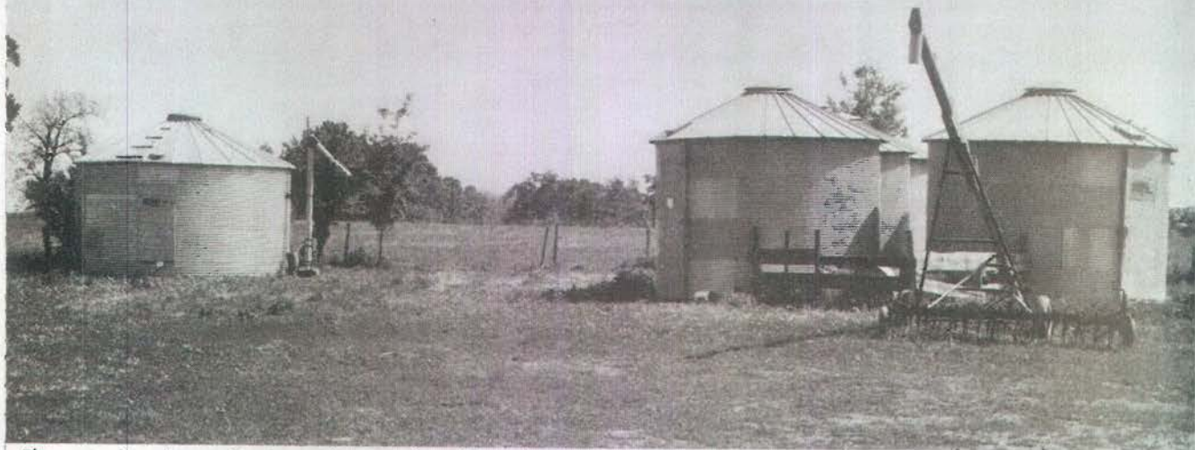
The overall system: Grain can be transferred from batch drying bin to other bins by use of a vertical auger, adjustable down spout, and portable auger.
