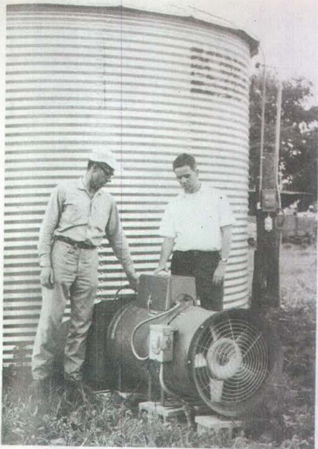
Matching air and heat is one of the desirable features of this installation. Mr. Roddy is pointing out his 3 horsepower fan and 210,000 BTU heater to Bob Kilburn, TVA Agricultural Engineer. Over or under-matching these can mean trouble and expensive time.
