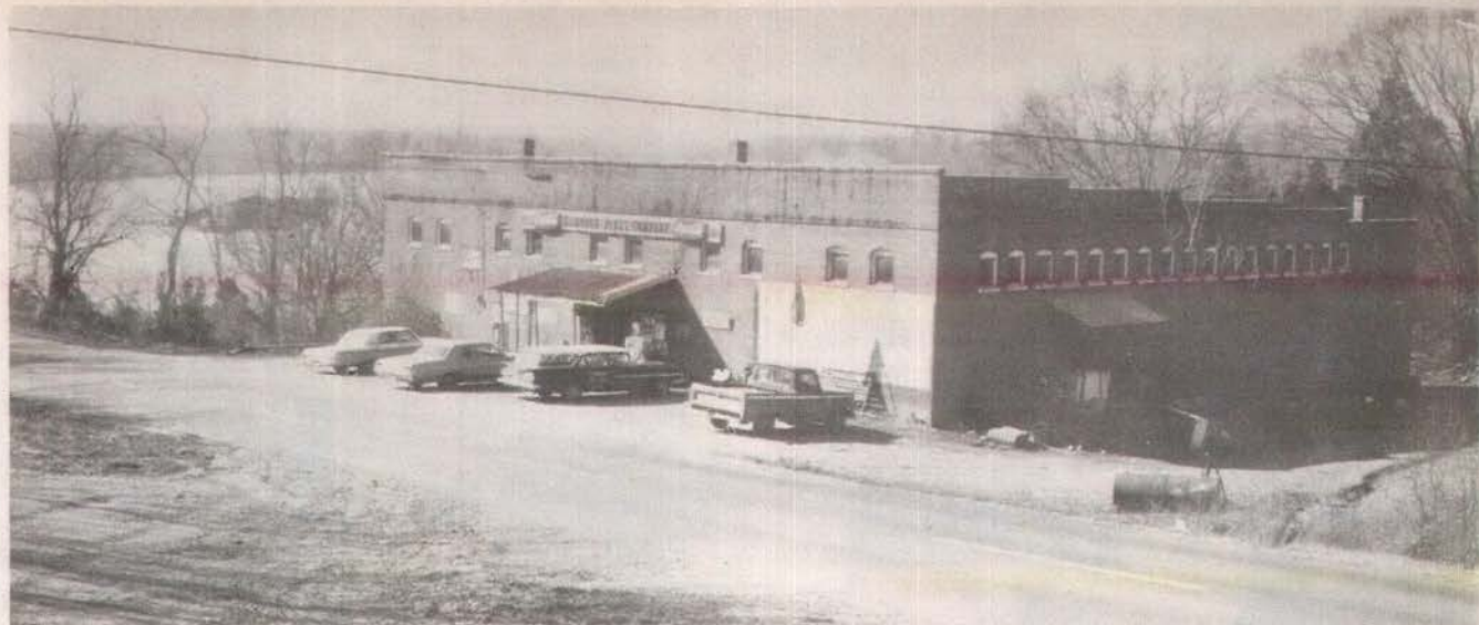
Harbour Pitts Store is nestled on the banks of the Tennessee River in the Cerro Gordo community.
