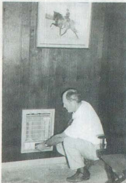
C. A. Bobo is shown here adjusting the thermostat on one of the 3,000-watt wall heaters located in his office area.
