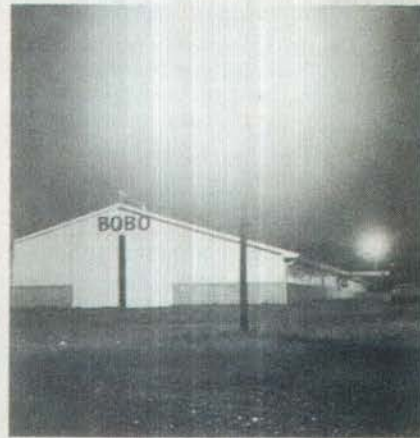
Four 175-watt mercury vapor security lights are evenly positioned around the Bobo walking horse barn. Each light is equipped with a photoelectric cell that automatically turns the light on at night and off in the morning.
