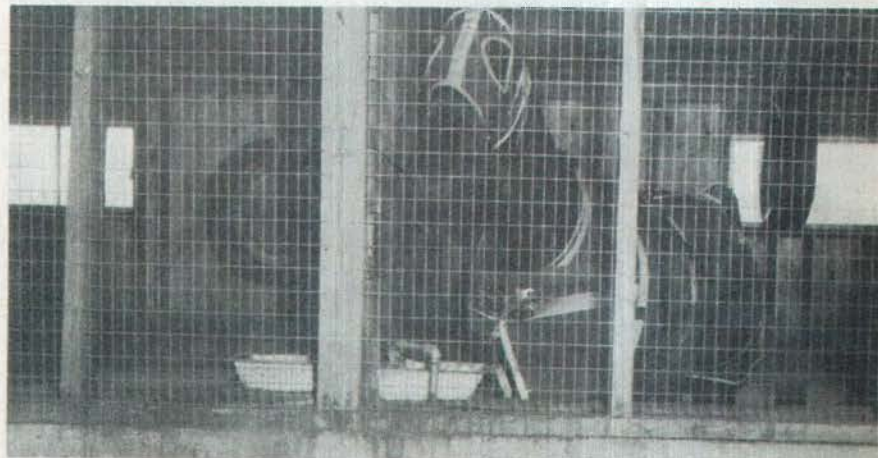
Water is supplied to each stable by a float-type water system.
