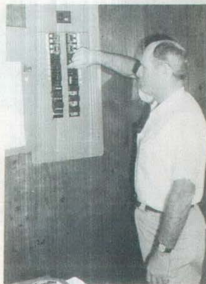
A 200 amp. main service panel adequately serves the electrical load and convenience outlets at the C. A. Bobo walking horse barn.
