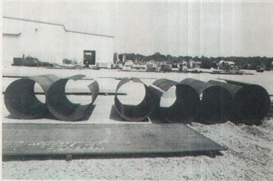
These air locks, sometimes called man locks, were rolled to this preliminary stage by Vanguard on its huge sheet metal roller. When completed, they will be used in underwater construction to get workers to underground work areas.
