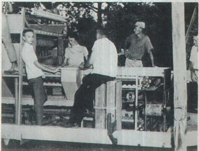
The pepper that is too green or has defective spots on it is culled and fed back to the cull sacks here. The good pepper is taken to the large truck by conveyor. Shown with the machine are Robert Nash, R. D. Clark, Fay Thacker, Jim Hockaday, and Jerry Campbell.
