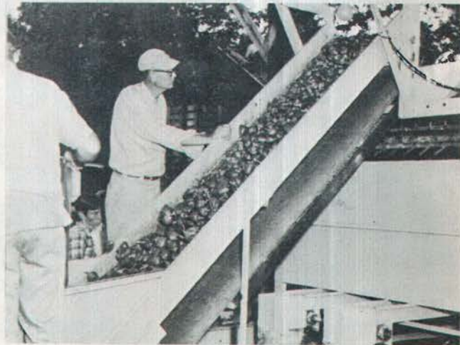
Estel Forsythe of Selmer, Tennessee is watching his pepper go through the grading machine. The pods that are too small, or are defective otherwise, are fed into the sacks at the bottom of the machine.
