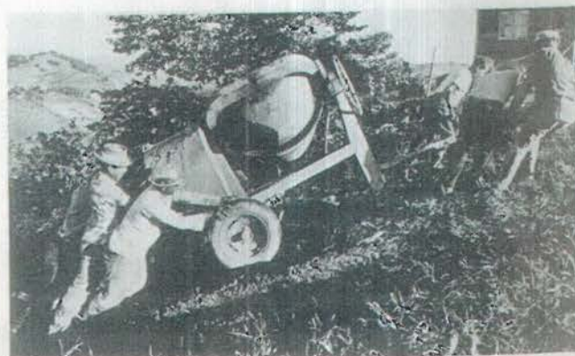
Rural workers at a do-it-yourself housing effort near Barranquitas, Puerto Rico, strain to move a cement mixer up a muddy hill.
