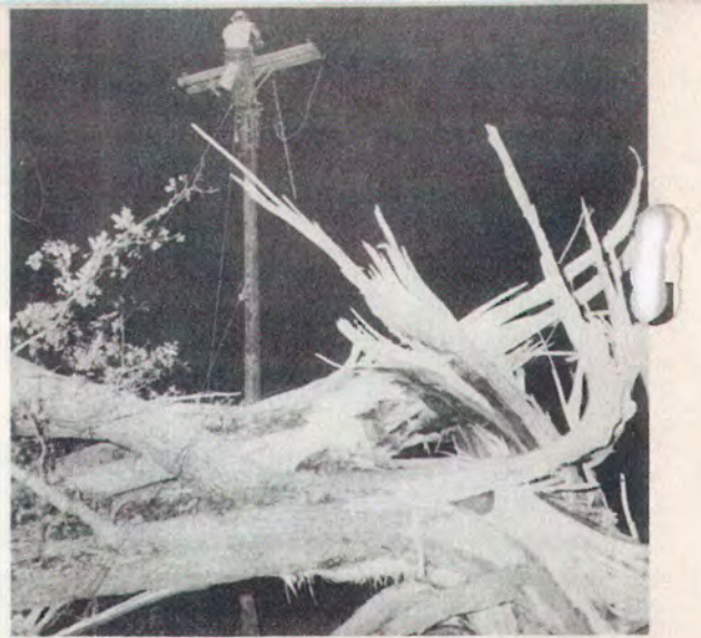
Splintered tree in Lewellyn community shows the strength of the wind, contributing factor to power outage. CEMC workman is atop pole in background.
