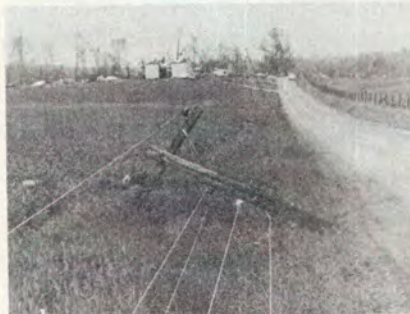
Twisted and broken pole in Robertson County shows the strength of the wind. Building damage shown in background.
