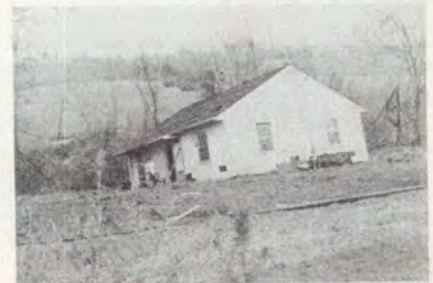
This house was completely swept from its foundation and set down some 200 feet down the hill.
