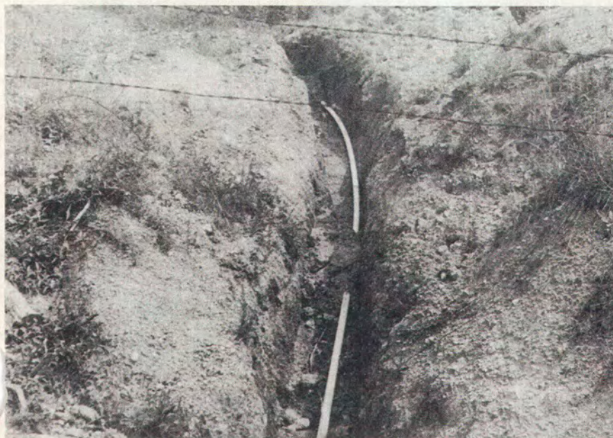
The 2½" plastic pipe was laid 24" underground along with the electric line which controls the pressure electrode.
