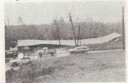
W. R. Edison chicken house on highway 76 was severely damaged and several hundred chickens were lost.
