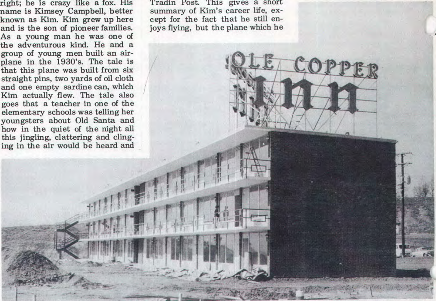
The Ole Copper Inn, as it appears going west on U.S. Highway I-64. The construction in foreground is the swimming pool.
