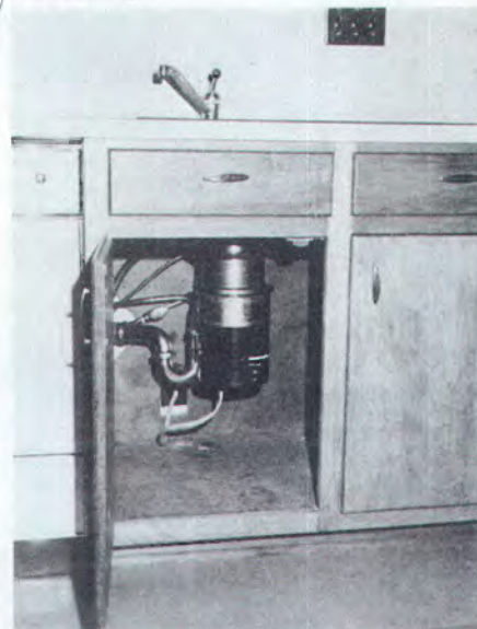
This picture shows how the garbage disposer looks under the sink. A disposer can be added under any sink. This picture was made in Middle Tennessee Electric's Lebanon meeting room.
