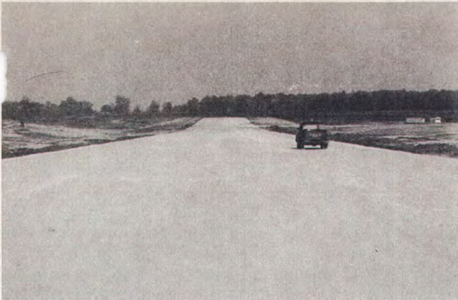
This new Smithville Municipal Airport runway, 3,400 feet long, is due for completion and the beginning of operation early this year.
