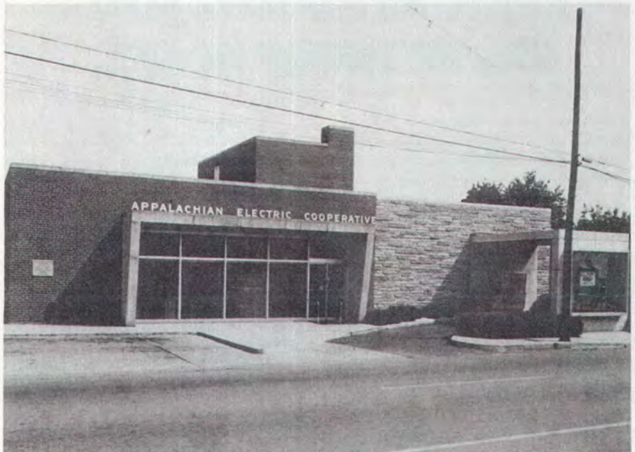
Appalachian Electric Cooperative, whose office headquarters at Jefferson City, Tennessee are shown above, has electrically served the Magnavox plant at Jefferson City since it was built in 1956.
