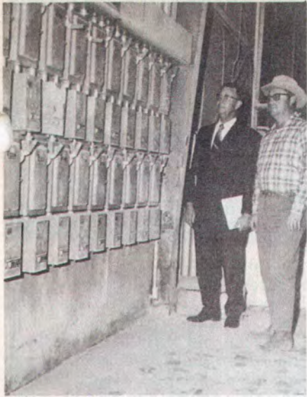
Control panel for the feed mill motors is well-designed and marked for convenience. Floyd Roberts of Gibson Co. Electric (left) and Gidcumb discuss the neat wiring job.
