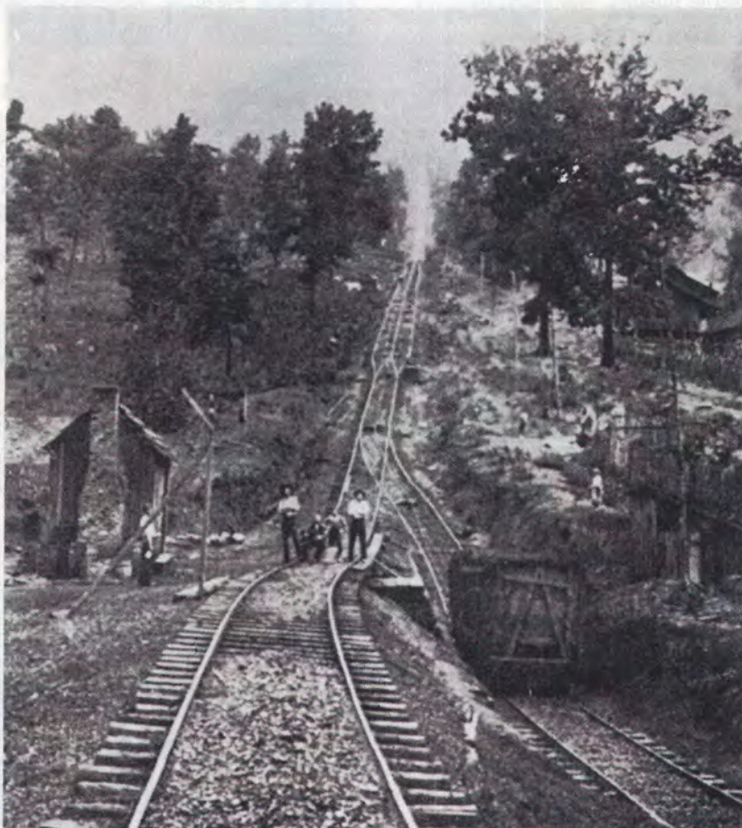
This picture of the Whitwell Incline appeared on the front cover of the Tennessee Products News in 1943. The Whitwell Incline was still in use at that time.
