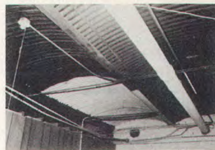
Beaver-board office partitions, drop cord lights, a steel roof and exposed steam pipes were prevalent in most of the Extension area in the Gibson County Court House basement prior to the renovation.
