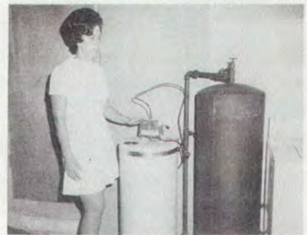
Mrs. Eugene Wheatcraft, above, of Hickory Hills solved her sulfur water problem with the chlorinator and filter. Her system was installed in the garage.
