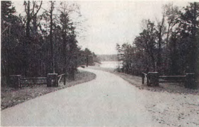
New streets have been laid out and surfaced. This entrance is the access to the picnic area.
