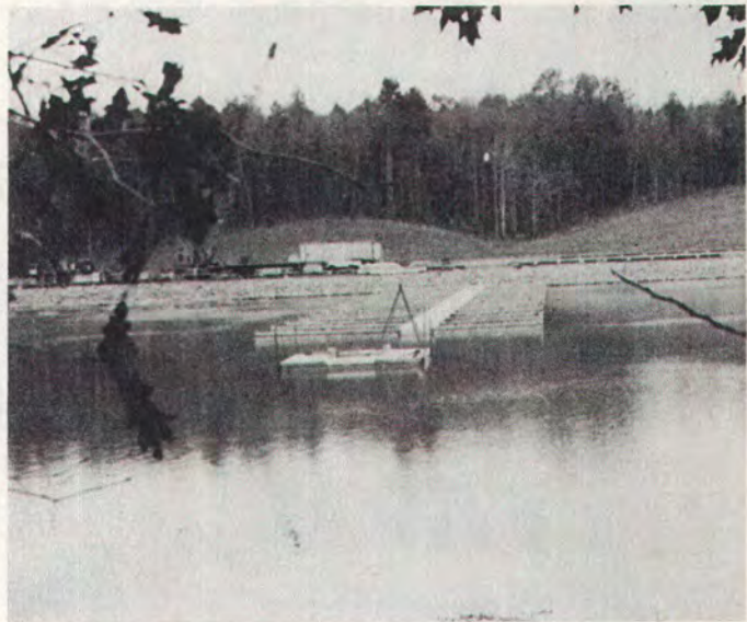
The apparent floating concrete marina will be one of the main gathering places. There will be 76 covered slips and a fuel and transit pier.
