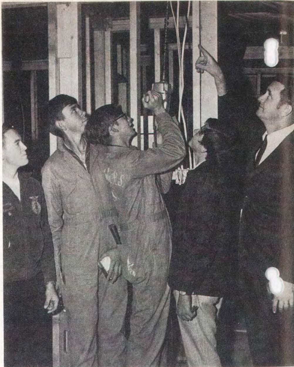
Jack Parnell, an Electrification Advisor of Gibson County Electric Membership Corporation, supervises a wiring installation being made by group of Lake County High School students on house under construction. Co-op electrically serves Tiptonville, site of Lake County High School. Boys receive two hours of credit each year toward graduation.
