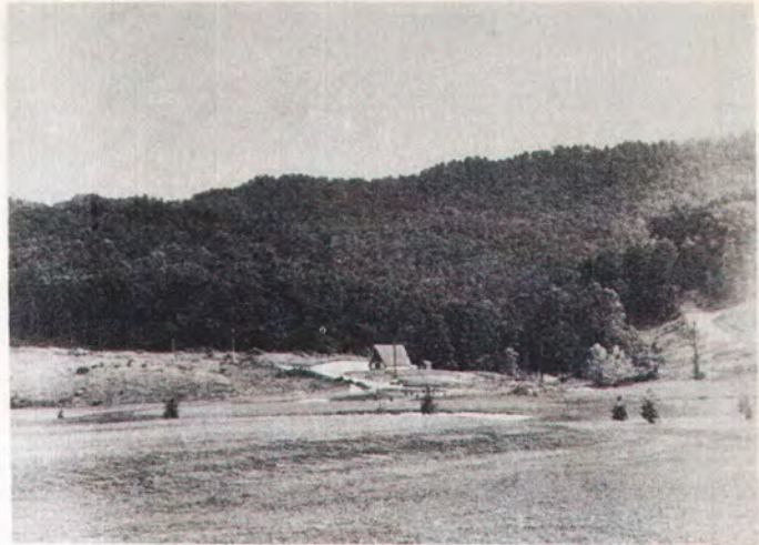
A view from No. 4 green looking northeast at the club house in background.
